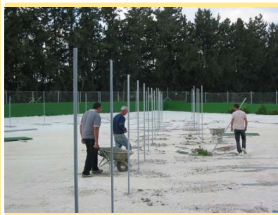
Erecting fencing posts for the exercise yards
